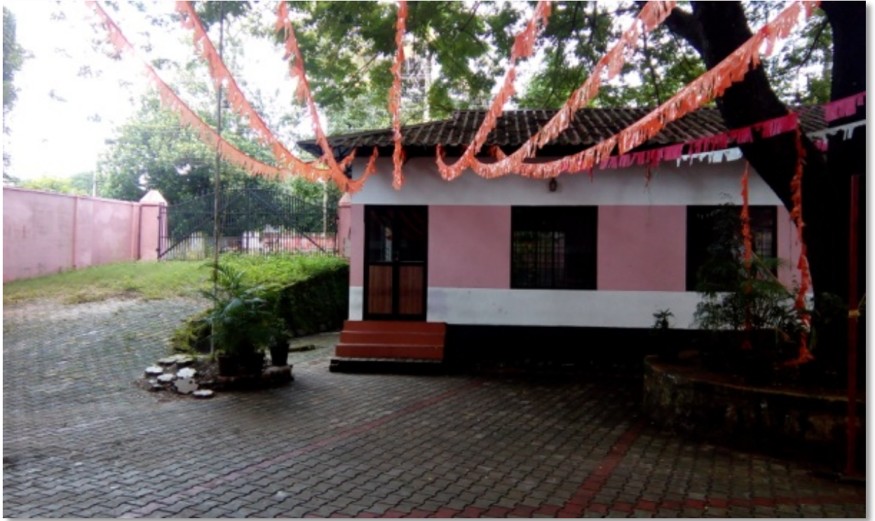
Figure 18: Compound Wall of Existing Campus
