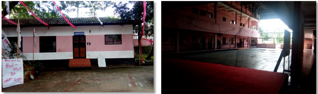
Figure 21: Existing Canteen and indoor court
