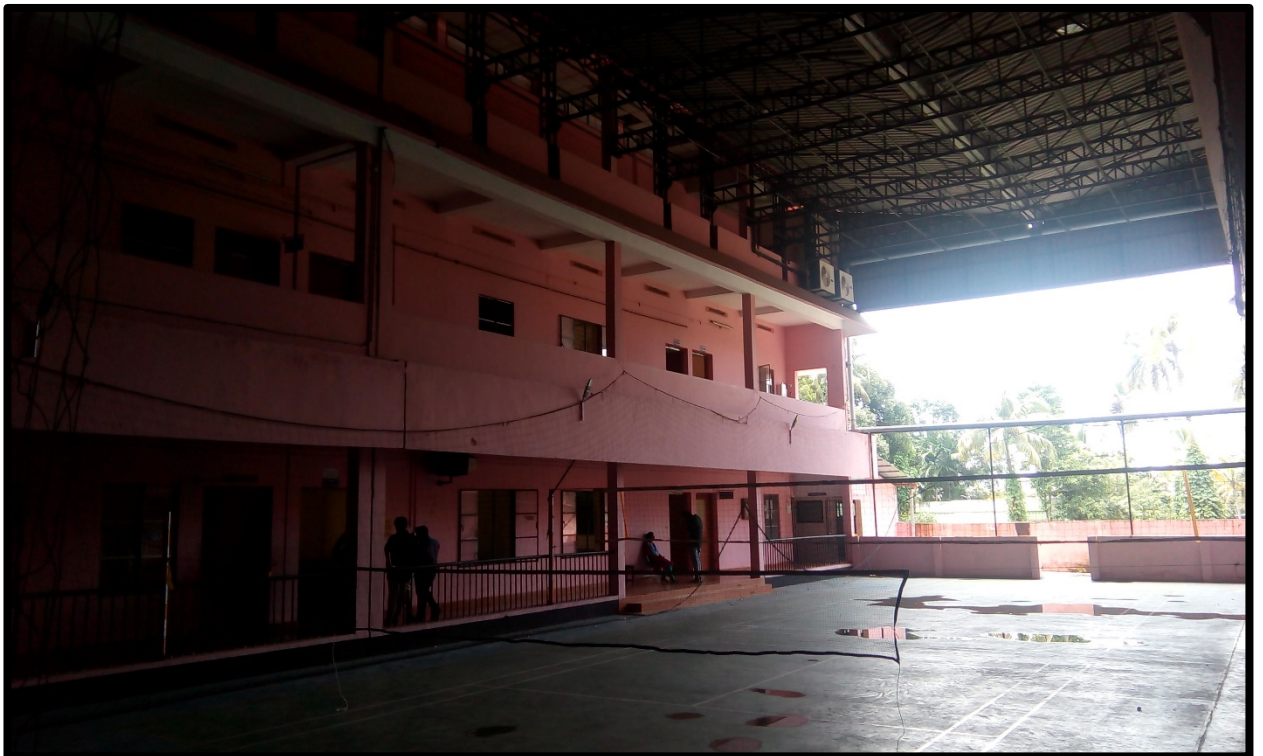
Figure 13: Existing indoor court
